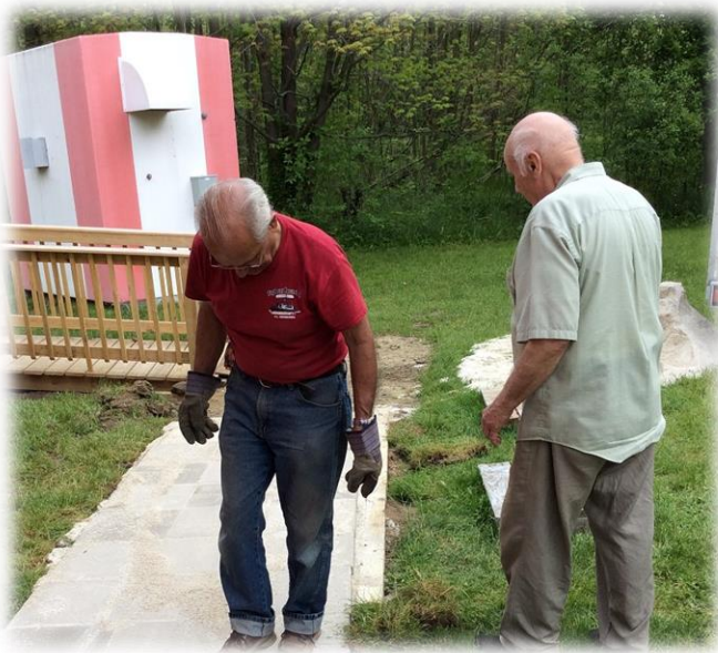
Joe and Gene laying blocks
