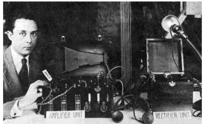
The “mousetrap” was a receiver for a radio amplifier that could run on AC. This was considered a breakthrough because at that time radios were only able to be powered by direct current (DC) provided by batteries. These batteries
